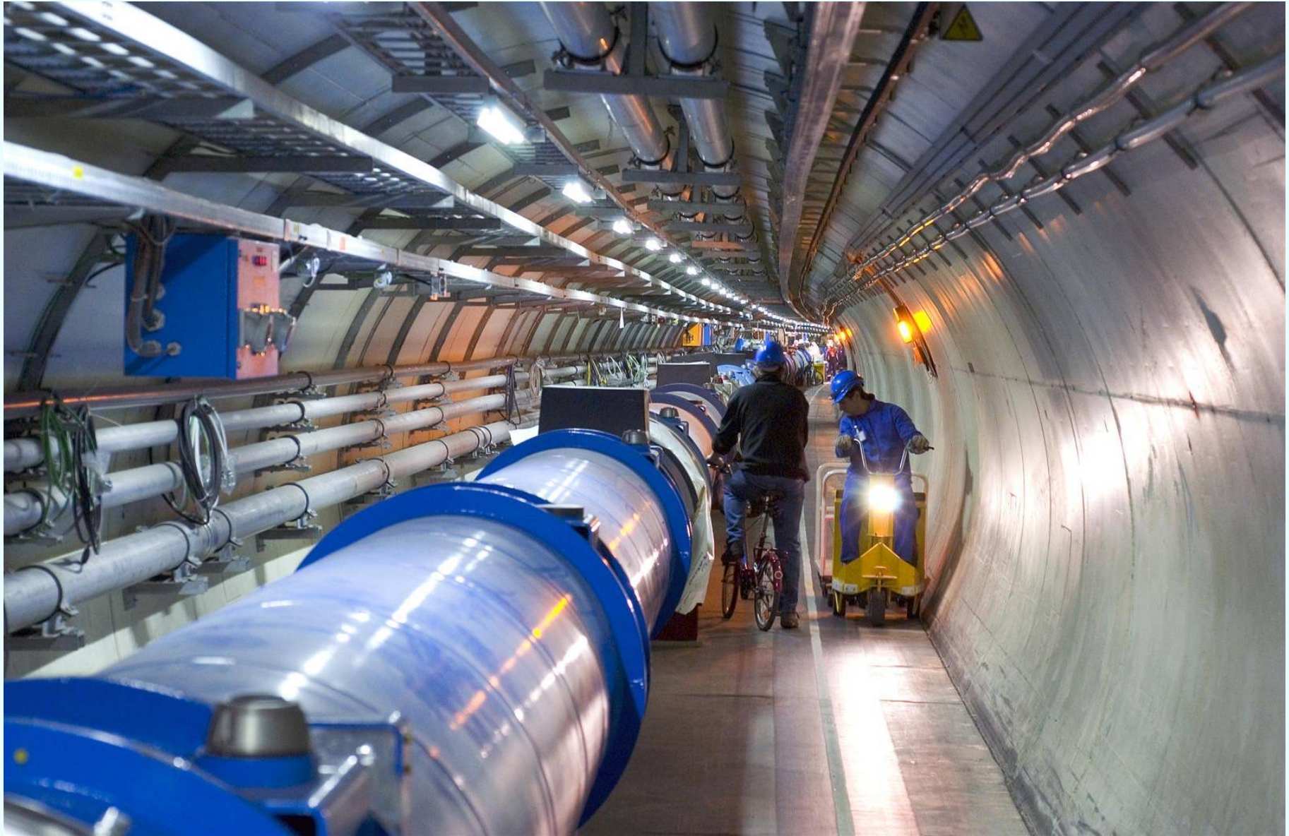
The LHC tunnel – with bending magnets as far as the eye can see
