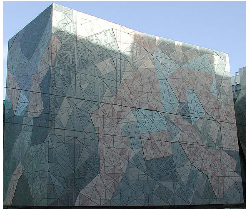
The Federation Square buildings in Melbourne, Australia
